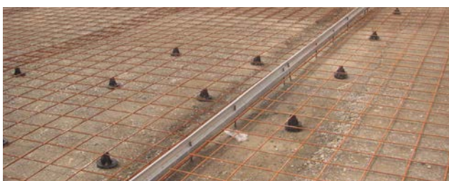
A continuous smooth joint between lengths of Keyjoint can be accomplished when joining clips are used.
